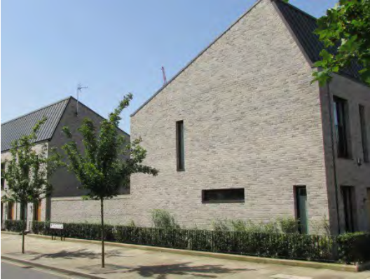
A distinctive roof profile using contemporary materials at Timekeepers Square, Salford
